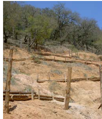
Ongoing restoration on the destabilized and eroding slopes of the Sierra Gorda Reserve to help restore and protect the watershed.
